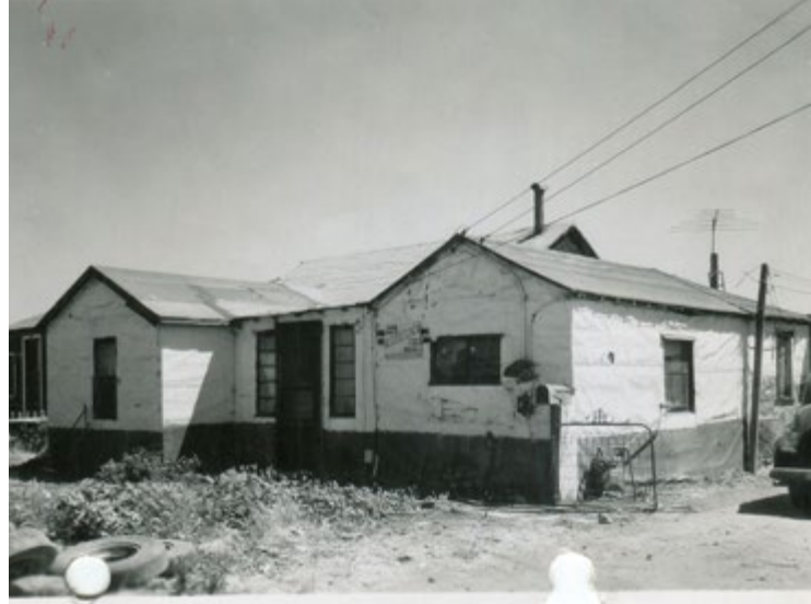
A small home with paper siding as well as a plywood roof. On the outside of the home is a sign that reads “For Sale.” Circa 1953. Photo courtesy of the Hayward Area Historical Society.
